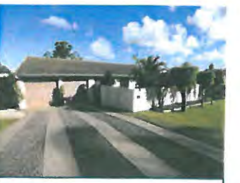
Permeable pavers like NDS Tufftrack are used as part of a residential stormwater system, allowing a permeable grass surface to be installed where an impervious hardscape was prior.
