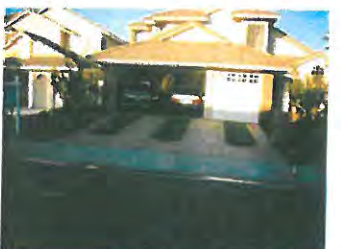
Permeable pavers like NDS Tufftrack are used as part of a residential stormwater system, allowing a permeable grass surface to be installed where an impervious hardscape was prior.
